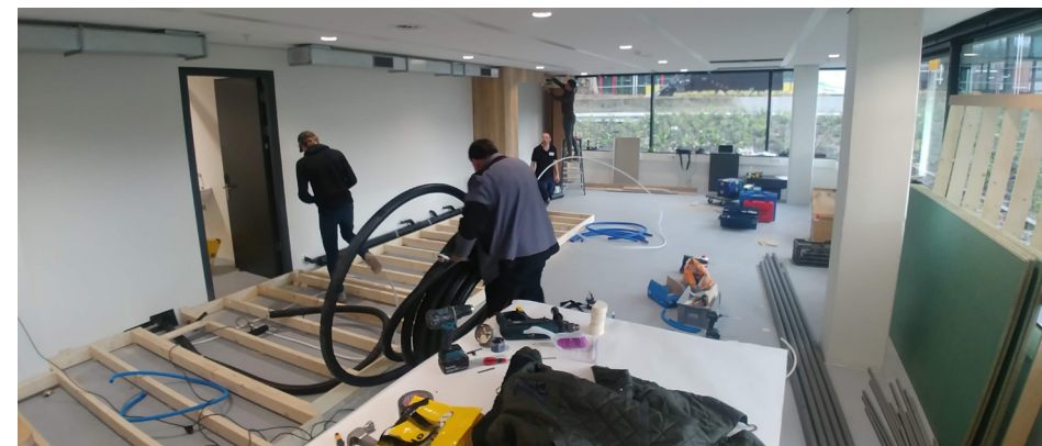
First day of Construction
